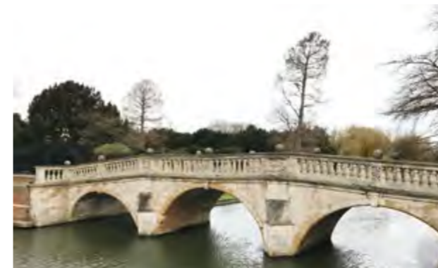
Clare College Bridge
